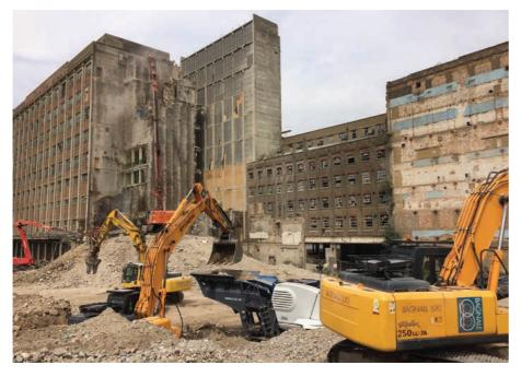
This allowed for a 47-tonne high reach excavator to be positioned over the tunnel at the rear of the site, with its 28m reach being used to take the building down floor by-floor, negating the need for any internal access by personnel.
